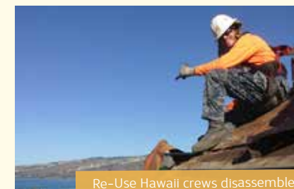
Re-Use Hawaii crews disassemble structures by hand.
