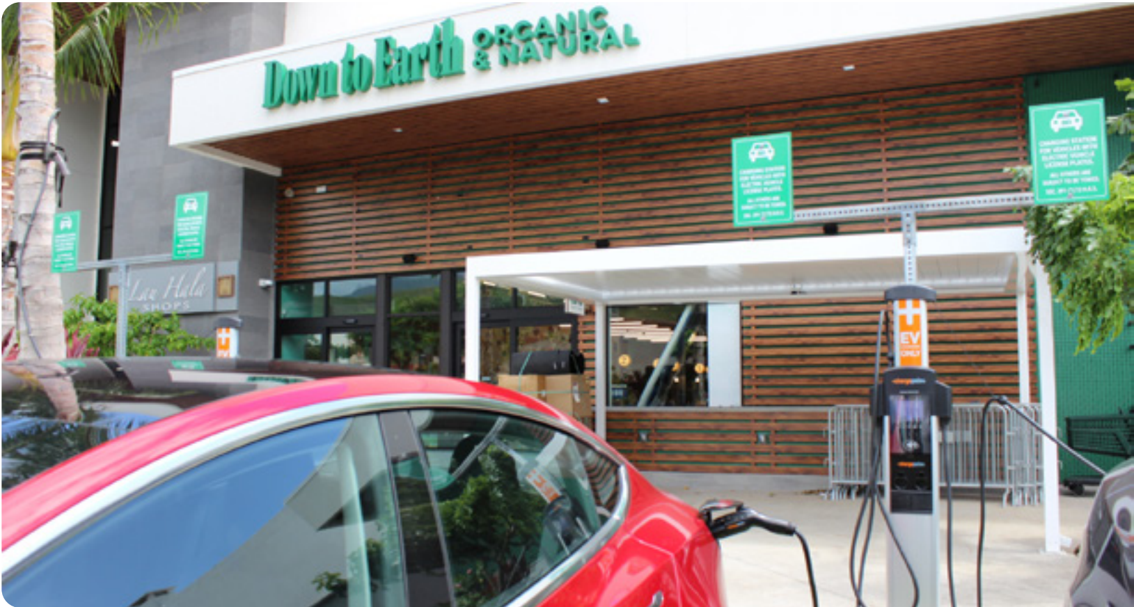
EV CHARGING STATIONS AT LAU HALA SHOPS
