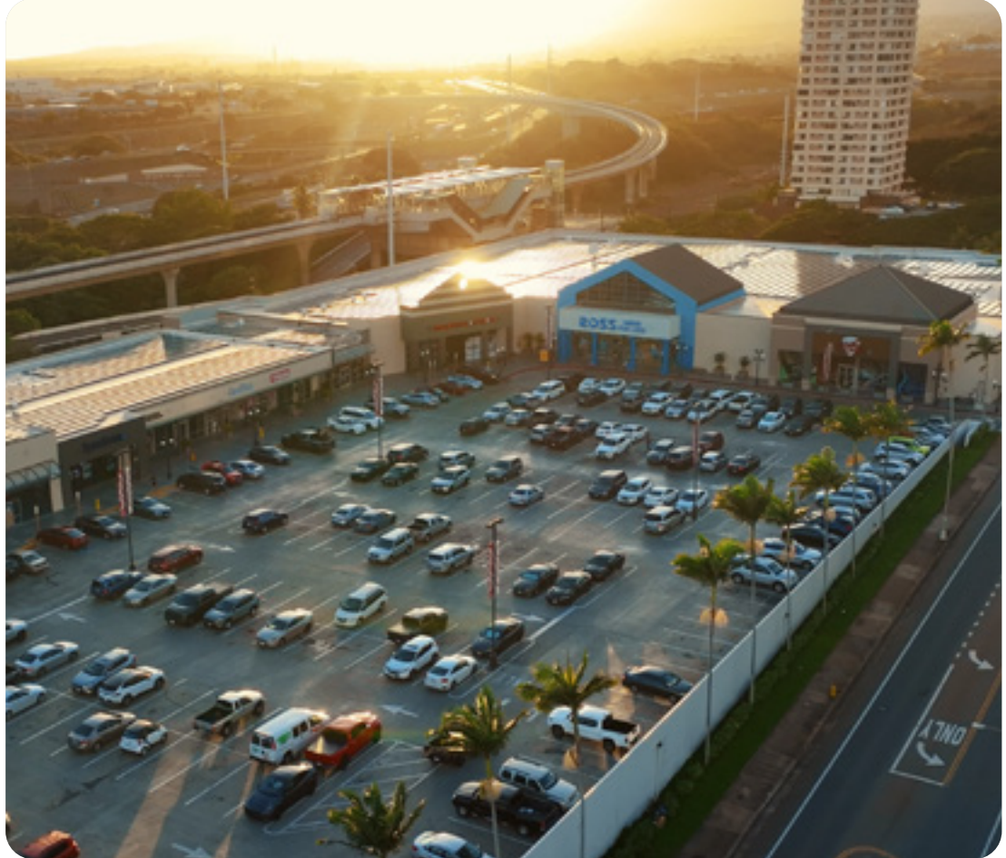
PEARL HIGHLANDS CENTER (PEARL CITY, O'AHU)
